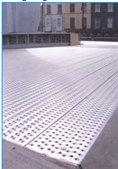
Exterior stage area with lighting on underside.
