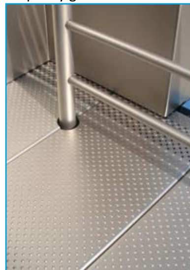
Exterior balcony with high quality glass bead finish.
