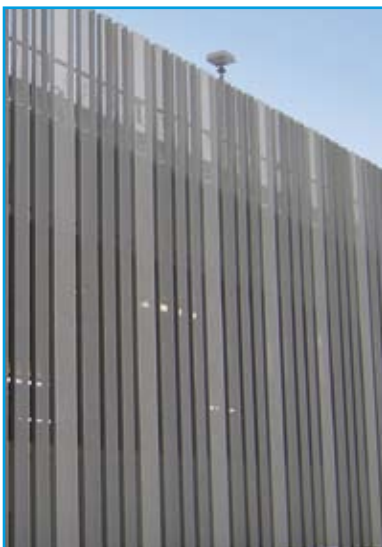
Car park cladding.
