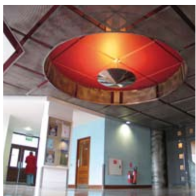
Perforated ceiling panels
