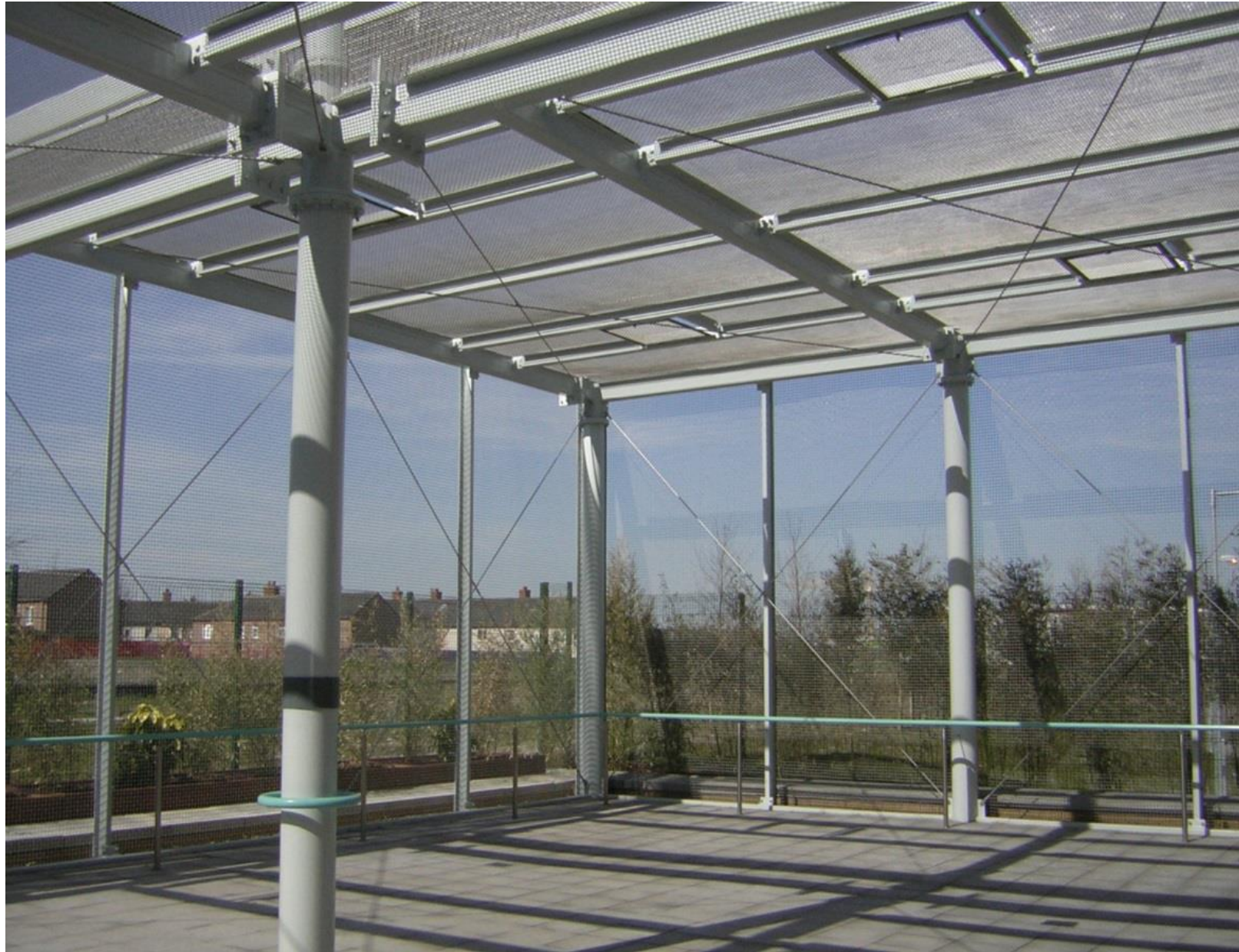
Woven Wire Mesh 12mm mesh in 4mm 316 quality stainless steel wire, security panels upon entrance to train station
